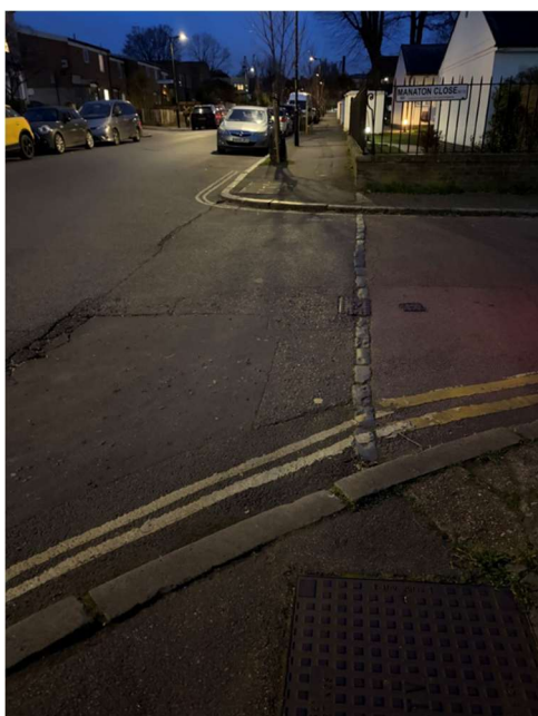
Figure 4-11: ATZ Route 4a – Worst Point (Night) – Lack of Tactile Paving and Dropped Kerbs at Crossing on Consort Road
