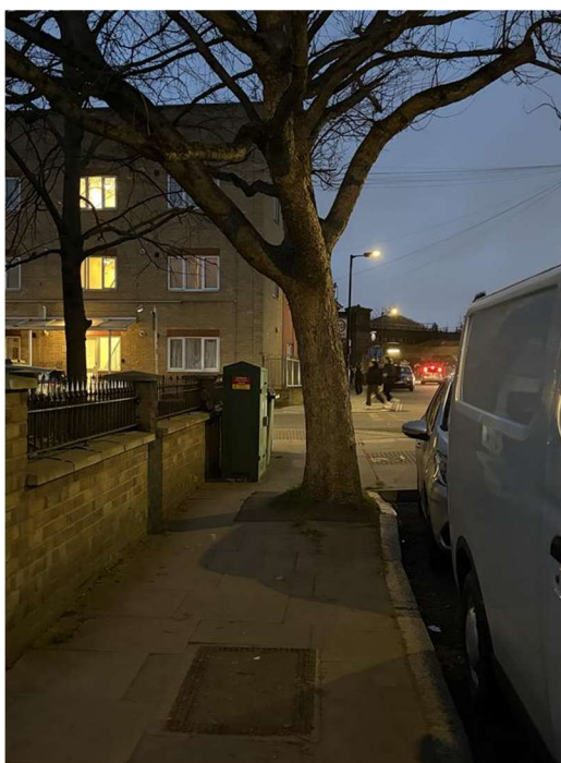
Figure 4-7: ATZ Route 2 – Worst Point (Night) – Narrow Section of Footway and Pinch Point on Southern Footway of Brayards Road Caused by Street Tree and Utility Cabinet
