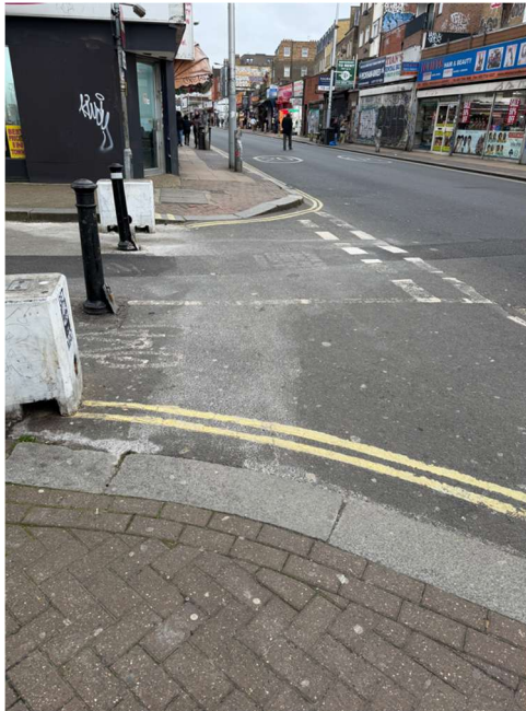
Figure 4-9: ATZ Route 3 – Worst Point (Night) – Lack of Tactile Paving and Cracked Paving Surface at Crossing on Rye Lane
