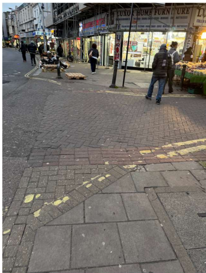
Figure 4-5: ATZ Route 1 – Worst Point (Night) – Lack of Tactile Paving and Inappropriately Positioned Bollards at Crossing on Rye Lane
