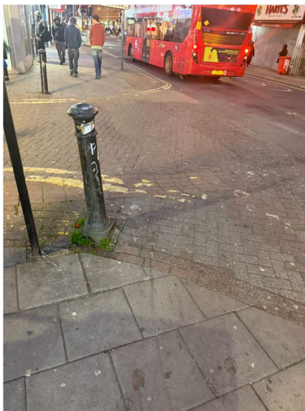
Figure 4-5: ATZ Route 1 – Worst Point (Night) – Lack of Tactile Paving and Inappropriately Positioned Bollards at Crossing on Rye Lane
