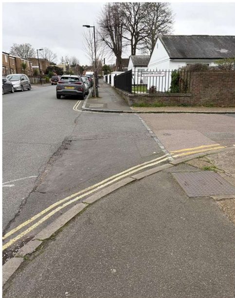
Figure 4-11: ATZ Route 4a – Worst Point (Night) – Lack of Tactile Paving and Dropped Kerbs at Crossing on Consort Road
