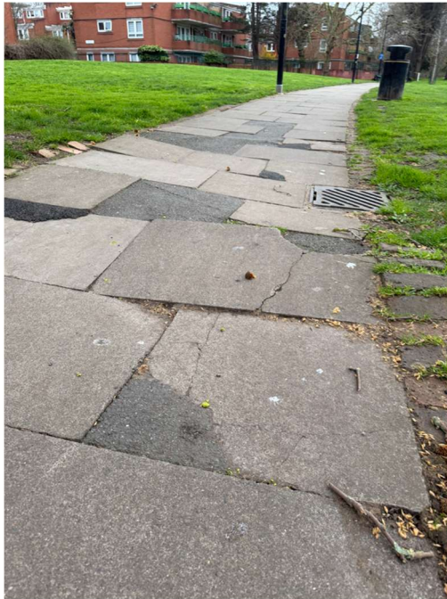
Figure 4-17: ATZ Route 6 – Worst Point (Night) – Cracked and Uneven Paving Surface along Shared Footway/Cycleway through Cossall Park
