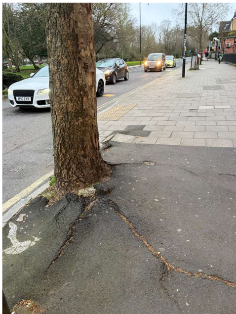
Figure 4-15: ATZ Route 5 – Worst Point (Night) – Cracked Paving Surface on Western Side of A2215 Peckham Rye caused by Tree Root Growth
