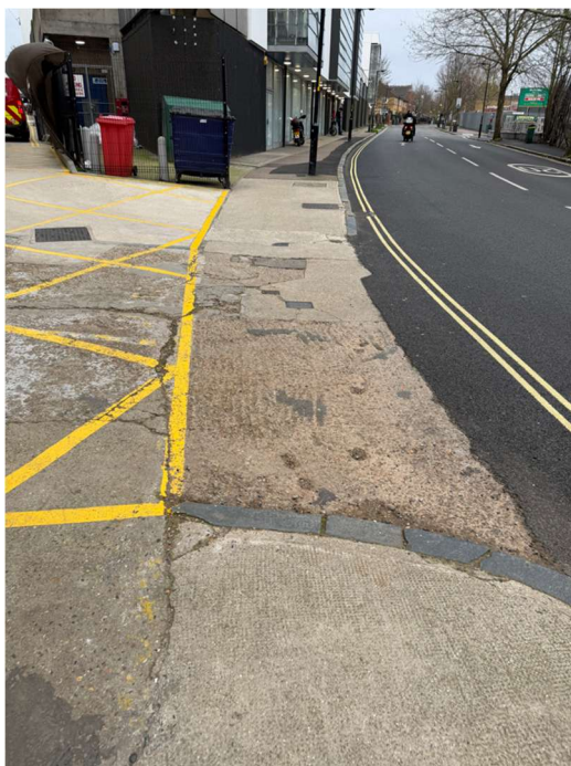
Figure 4-19: ATZ Route 7 – Worst Point (Night) – Lack of Tactile Paving, Cracked Paving Surface and Lack of Edge Definition on Western Side of Vehicle Crossover on Consort Road
